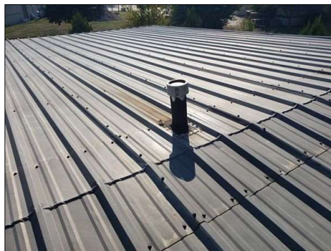
Chimney corroded
