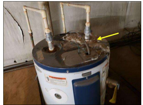
View of water heater, leaking
