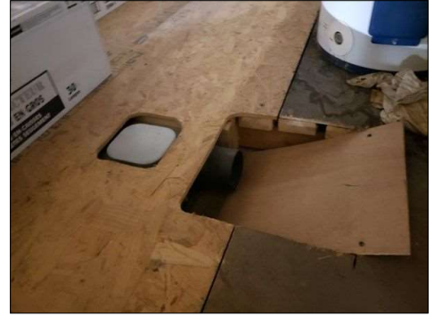
Restroom exhaust fan not vented to exterior
