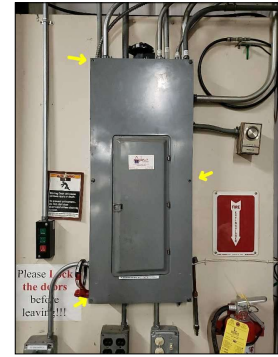
Missing fasteners
