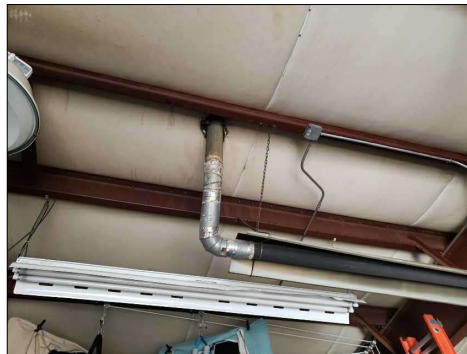
Corrosion on vent line
