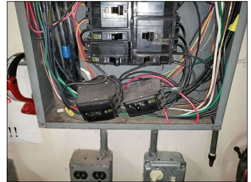
Improperly terminated wiring
