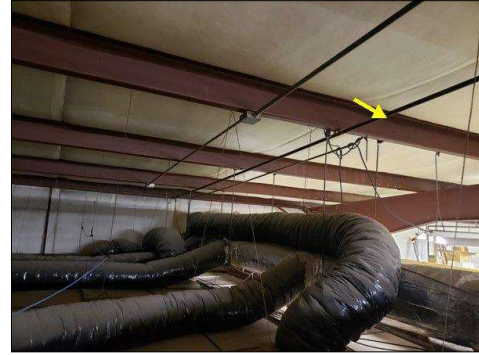
Gas line not properly marked
