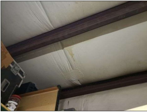
Moisture staining, past repair
