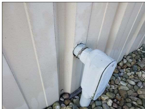
Utility lines need to be caulked where they enter the building
