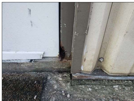
Damaged to door trim, gaps
