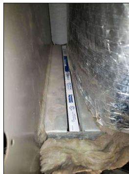
Furnace filter location.
