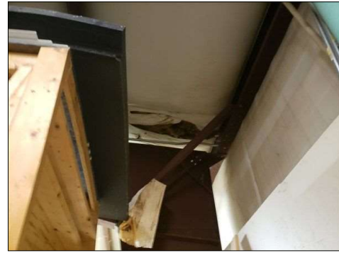
Moisture staining, damage to insulation
