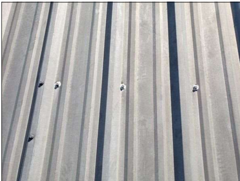
Fasteners have signs of past repair
