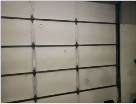
Damaged panels
